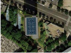
General view of the project
